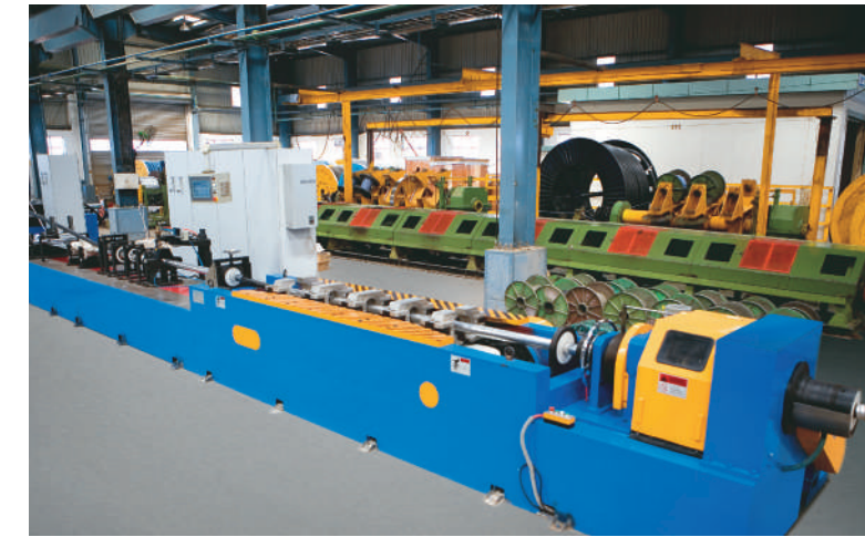
Aluminium Corrugation Sheathing Line
