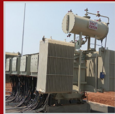
Inverter Duty Transformers
